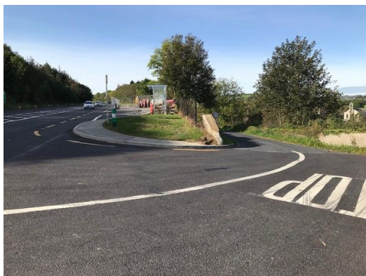
Figure 2-11 - Side Road with Acute Angle & Steep Approach and Typical Local Road Cross Section
